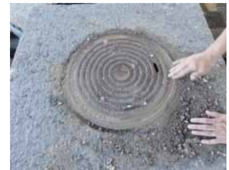
Material under Kellogg Street Bridge
