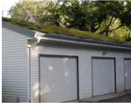
Green roof on resident's garage
