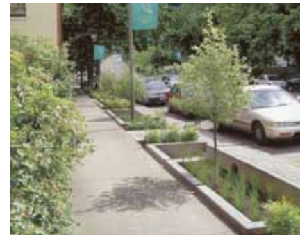
Portland Storm Water Planter, Portland, OR
