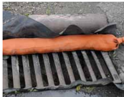
Construction site on East Side of St. Paul
