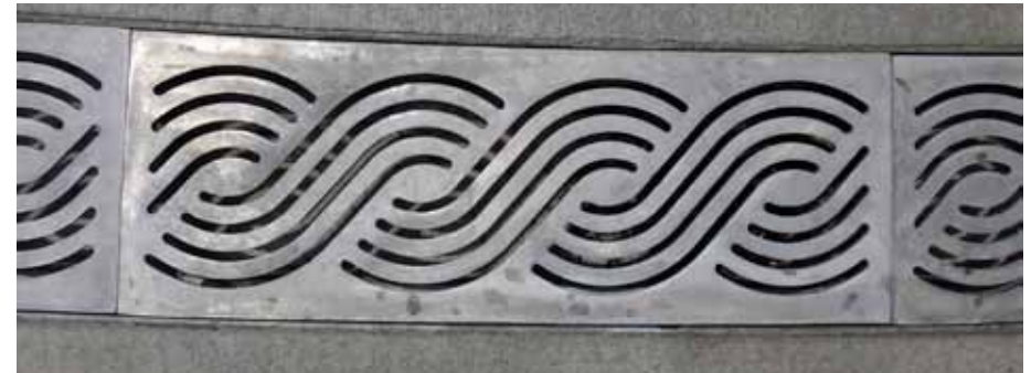
Grate, Roseville Library
