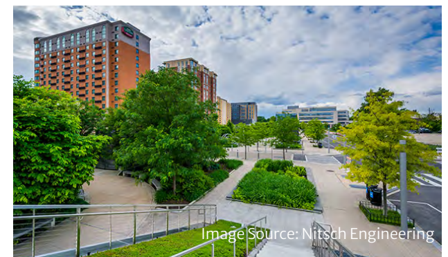
Canal Park district stormwater system - Washington DC
